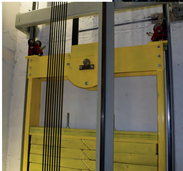
Counterweight with retained fillers
